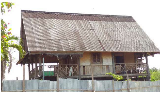
Photo 7: The only Stage House belonging to the late H. Anwar family and standing upright over some of the displaced villages. A zinc fence protects this cultural site from being damaged by irresponsible hands (Source: author’s photo 2018).
