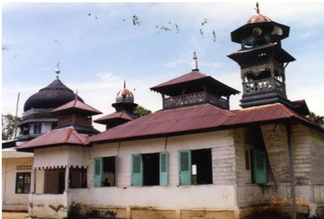
Figure 4. Photograph of Gunong Kleng Mosque in 2006 (Kemdikbud, 2015)
